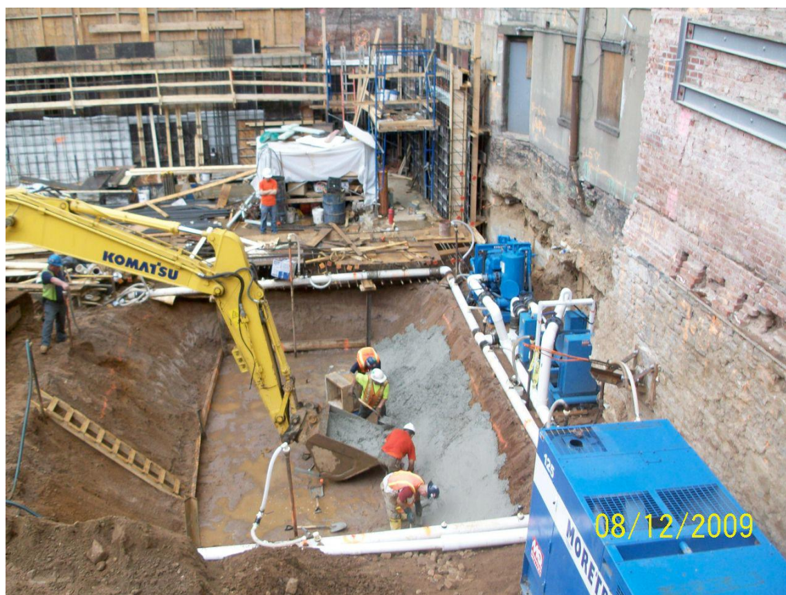
Figure 15: Display the Dewatering System
