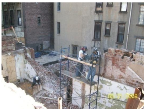
Figure 3: Shows Hand Demolition method being utilized
