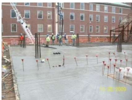
Figure 6: Pump Truck Placement Method
