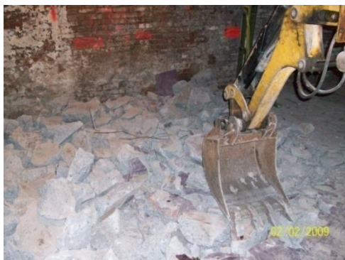
Figure 2: Shows an Excavator in the Demolition Phase
