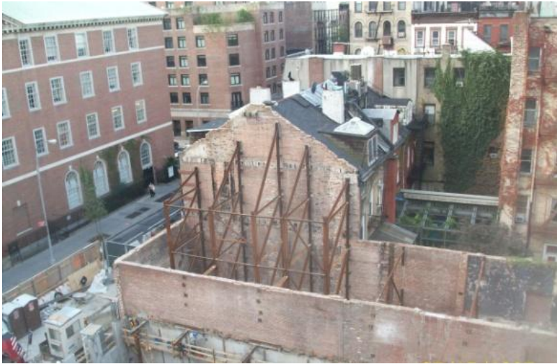
Figure 4: Shows Temporary Structural Steel Bracing
