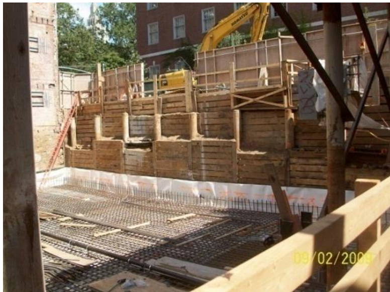
Figure 8: Shows the Sheeting (Lagging) and Piles on the East Side (Mac Dougal Street)
